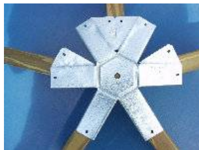
Figure 11: Pentagonal connection [12]
