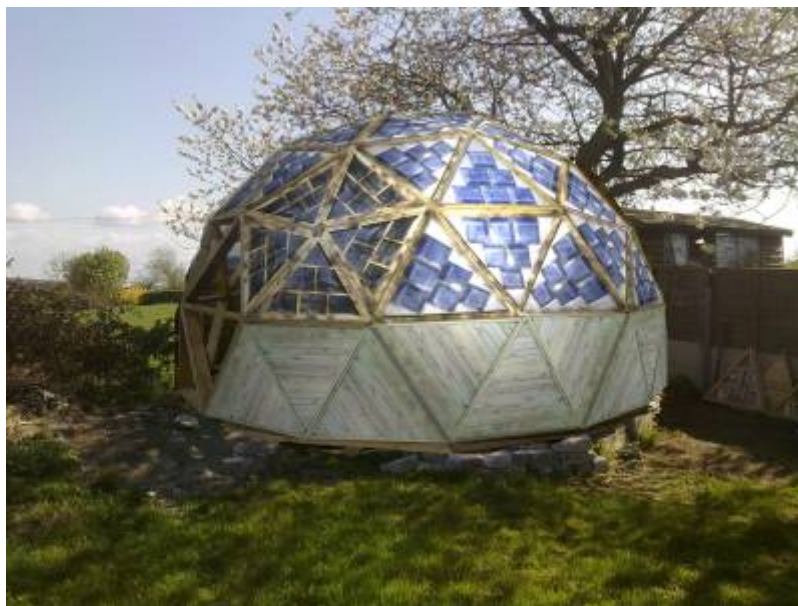
Figure 66: Solar panel on the dome [61]
