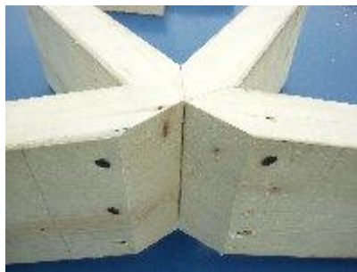
Figure 6: Angles at the end of a beam Dome kits, 2016. [6]
