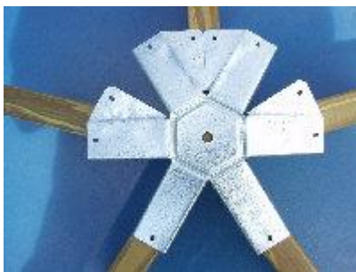
Figure 11: Pentagonal connection [11]
