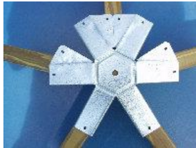
Figure 11: Pentagonal connection [11]
